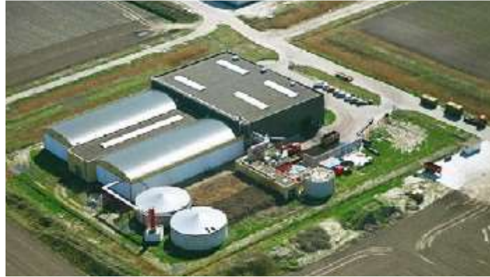
Figure 21. Biocel leach-bed batch digester facility in Lelystad, Netherlands From the Orgaworld website, accessed September 2007.
